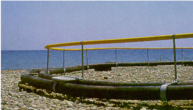
Powerring Mk II during erection in Cyprus
